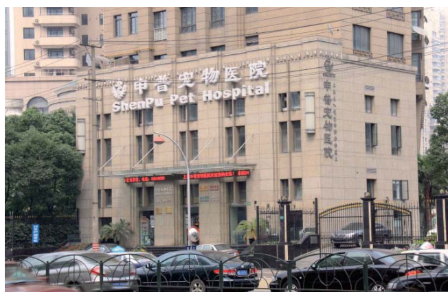
DATA Facility name: Shanghai ShenPu Pet Hospital Location: Shanghai, China
