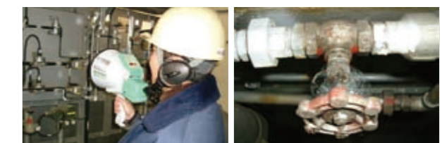
Checking that no air is leaking, using an air leakage monitor. Identifying the site of the leak using soapy water
