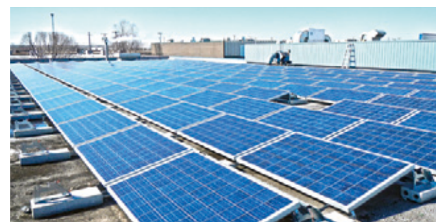
Top: Opening ceremony held on April 20, 2012 Bottom: Solar power generation facility capable of annual output of 60,000 kWh
