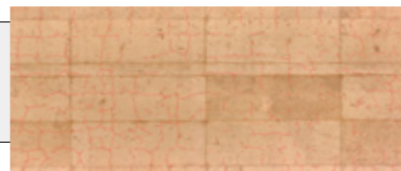
Take photographs of the concrete surfaces of bridges, piers, and tunnel for inspection. Upload the photographs to a server, and the service automatically detects highly precise images of cracks larger than 0.1 mm wide (shown as red lines). The service then automatically creates CAD data of images and crack detection results.
